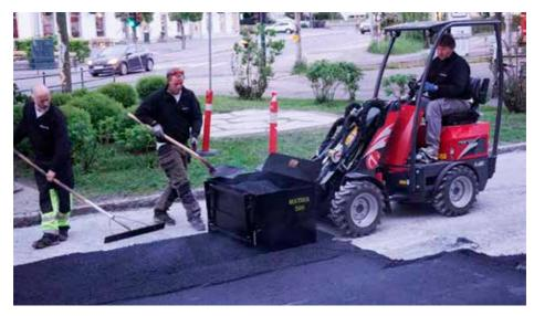
For smaller asphalt paving areas. The height of the asphalt layer can be adjusted manually. Also works well when distributing an even base for laying a brick or stone driveway.
